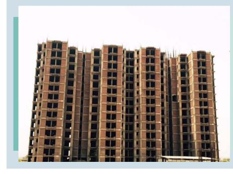
Towers A5, A6 Structure and Masonry work complete.Internal plaster till 12th floor done.
