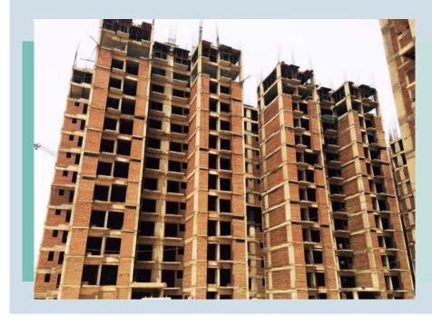
Towers B1, B2 B1- 12th floor roof casted and Masonry work complete till 10th floor. B2- 11th floor roof casted and Masonry work complete till 10th floor.
