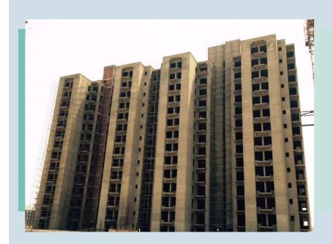
Towers A1, A2 Structure work complete. External Plaster front facade.
