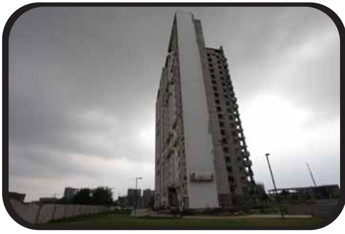
← Tower 5 External painting nearing completion
