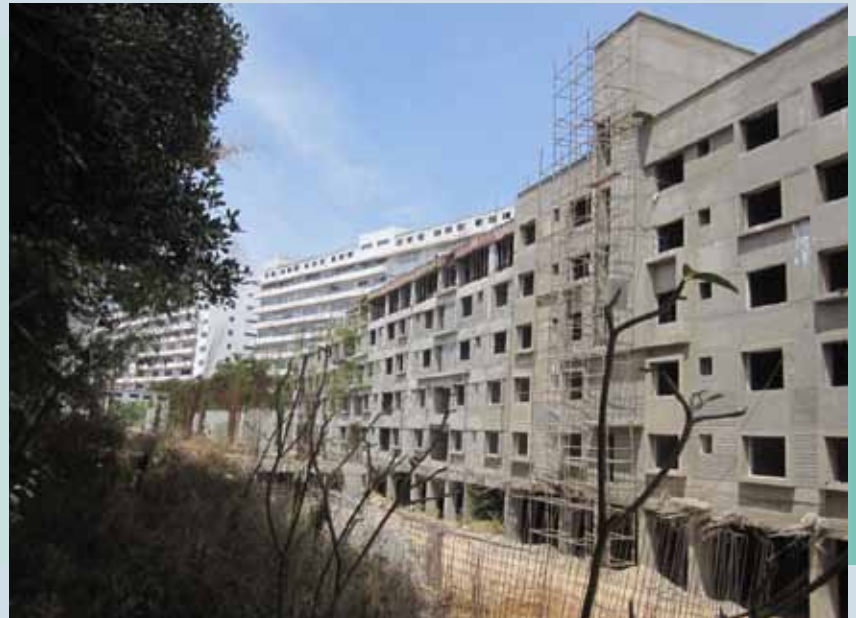
Work in progress for Tower 66 to 74
