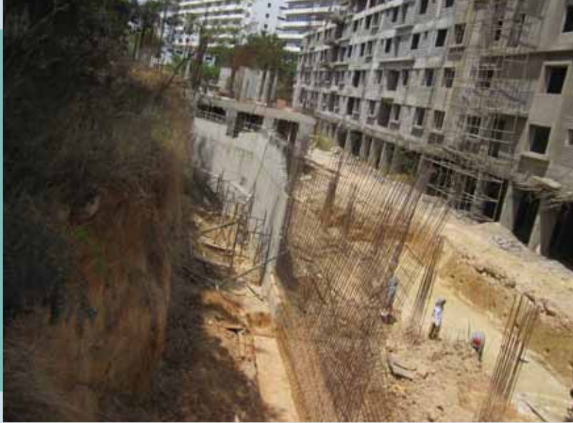
Basement ramp work in progress
