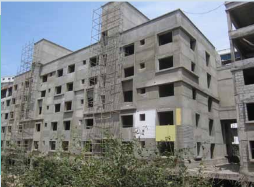
External plaster in progress for Tower 69 to 70
