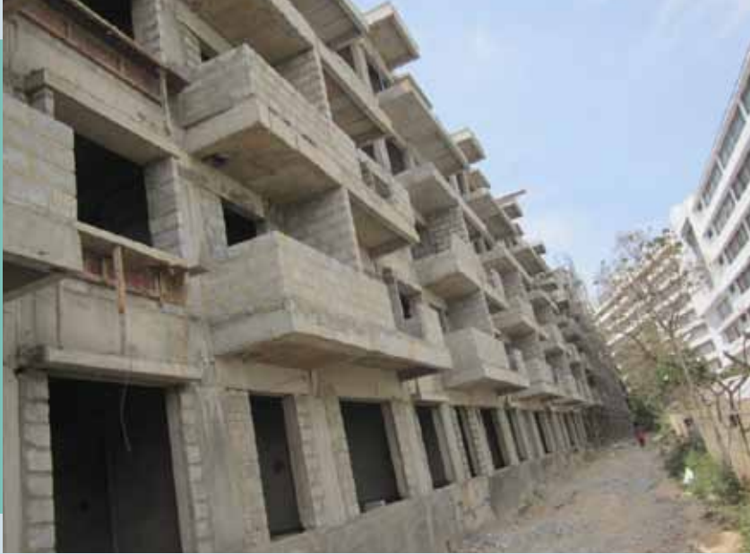
Work in progress for Tower 66 to 74
