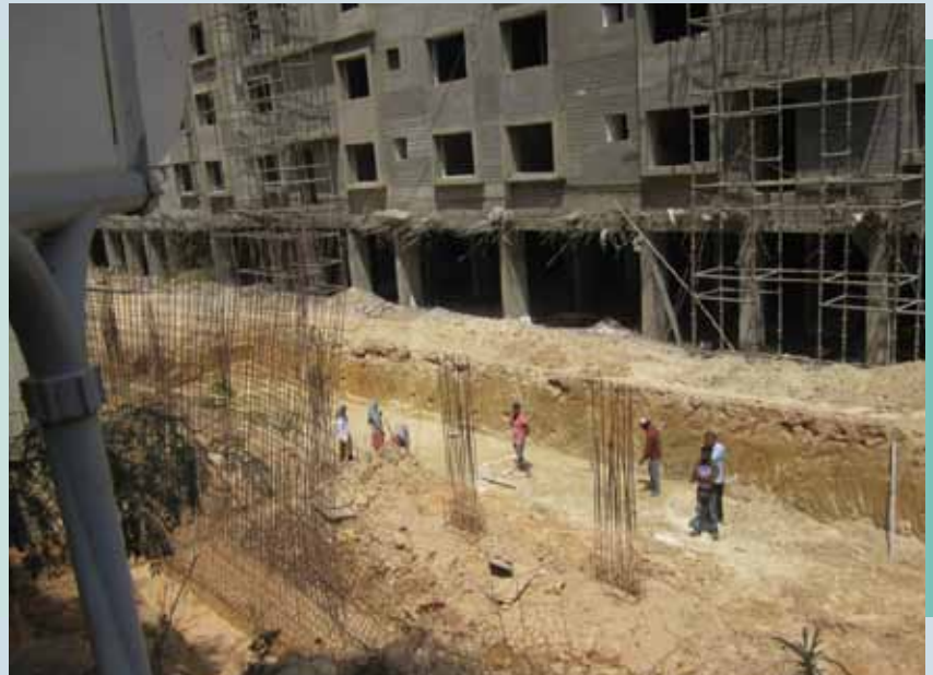
Basement ramp work in progress
