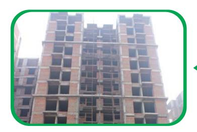
**Tower A3**Civil structure completed & masonry work in progress
