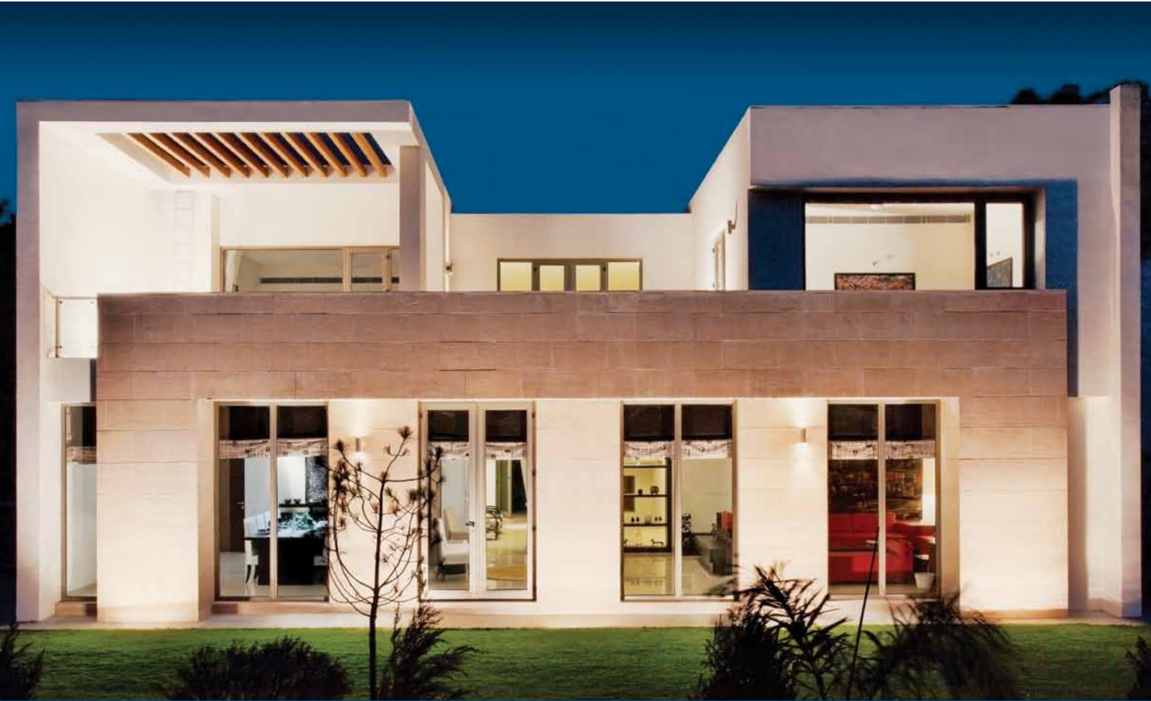
100% power back up
